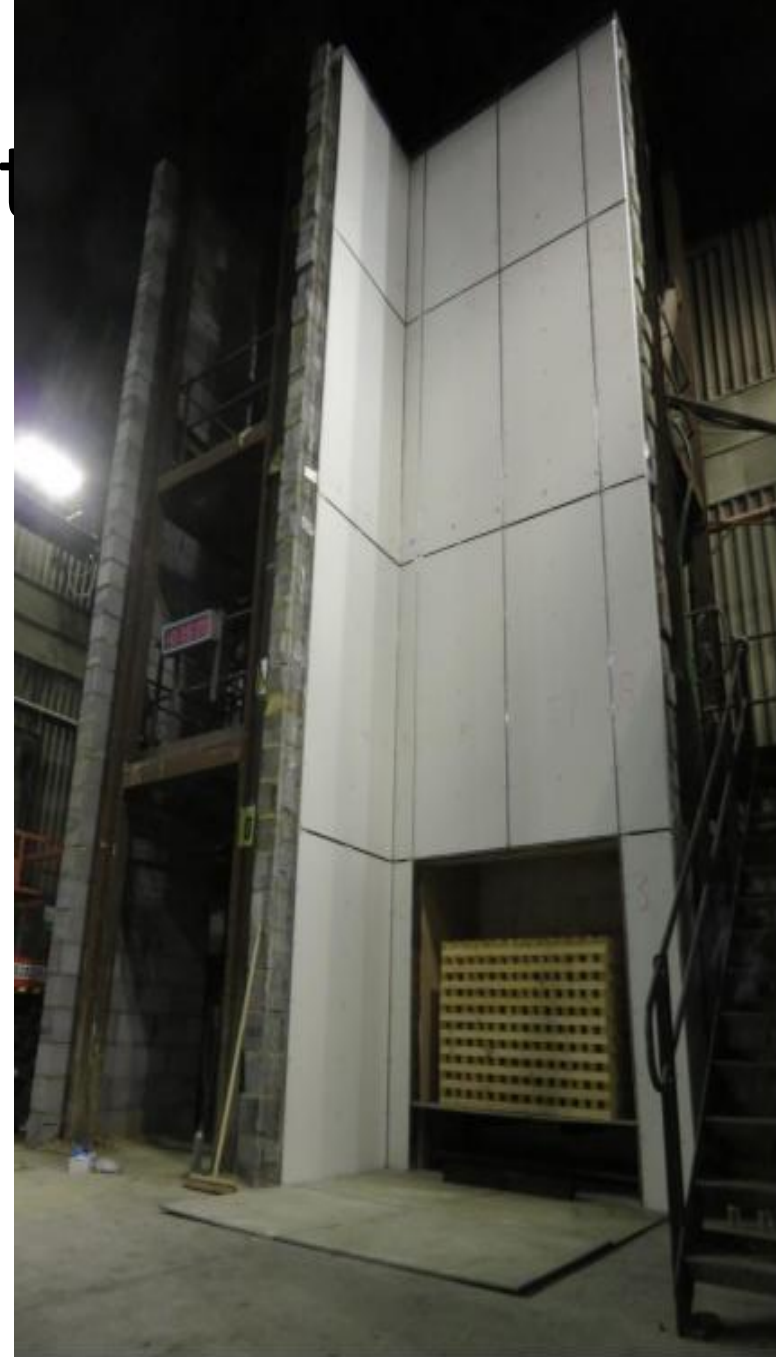
Figure 11. Completed installation prior to test.
