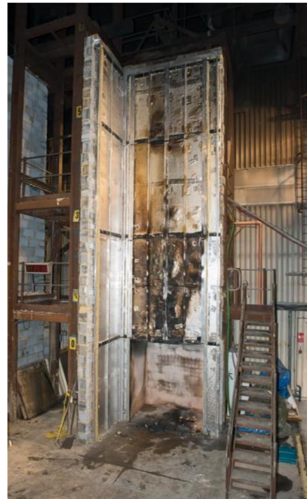
Figure 27. Full height photograph of system following removal of ACM panels.
