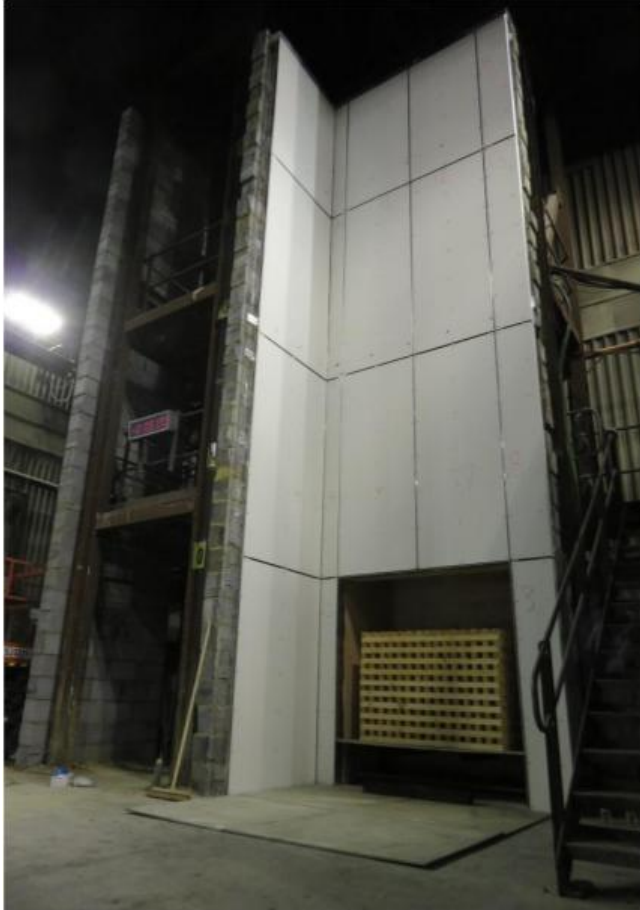
Figure 11. Completed installation prior to test.
