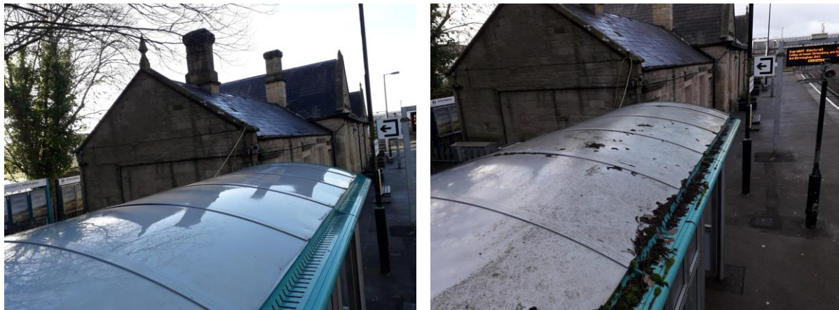
Deep clean of shelters at Ruabon as part station refresh
