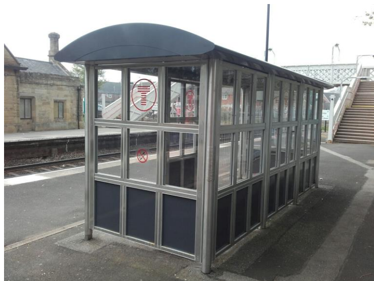
Refurbished platform shelter at Bridgend as part of Station Facilities and Rebrand programme
